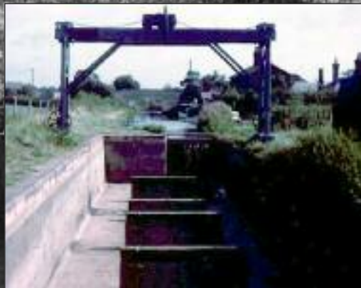
Lock one, Newport Canal. Converted into a dry dock is actually the start of the Newport Canal. Photograph taken in 1959 from the collection of © Tony Clayton.
