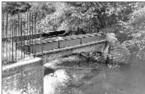
An aqueduct carrying a stream over the Shrewsbury canal at the foot of the Trench incline plane
