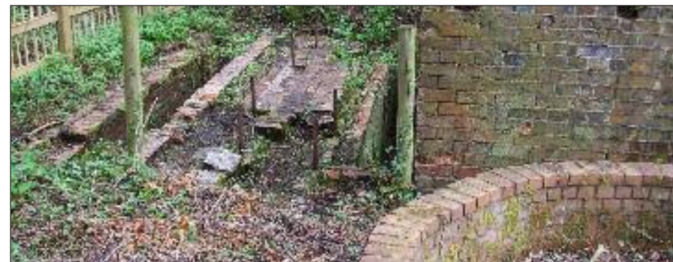
The remains of the winding house, pump mountings and flywheel pit
