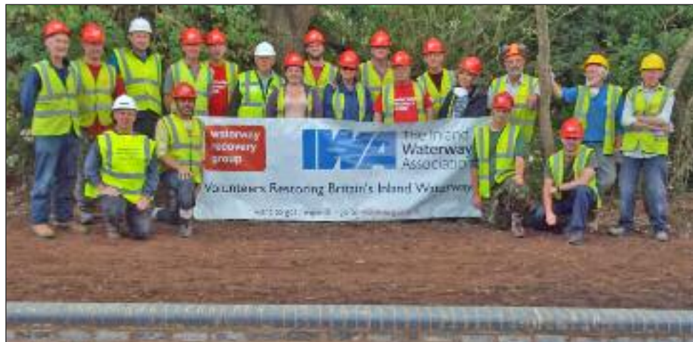
Members of the Waterway Recovery Group and the SNCT gather at Meretown Lock after finishing work
