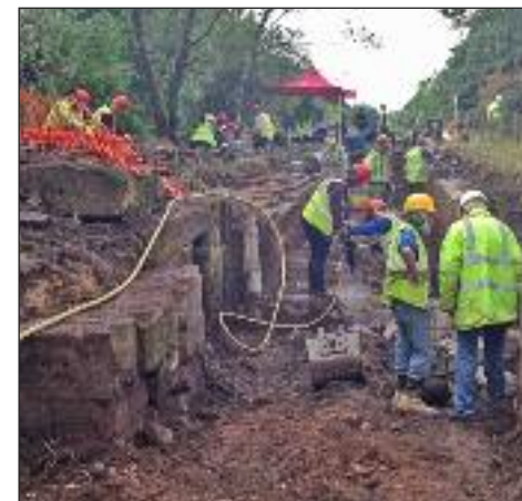
WRGies clearing concrete from the lock entrance with a jackhammer
