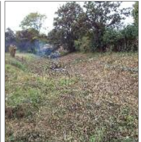
Clearance work at the Forton Bridge section
