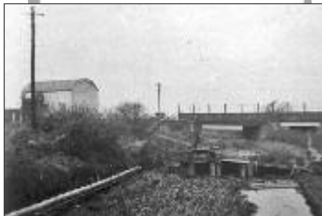
The Trench railway bridge over the Shrewsbury Canal in 1954
