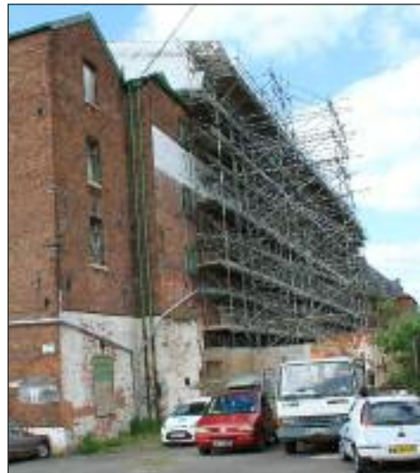
Exterior of the mill with scaffolding erected for earlier roof repairs
