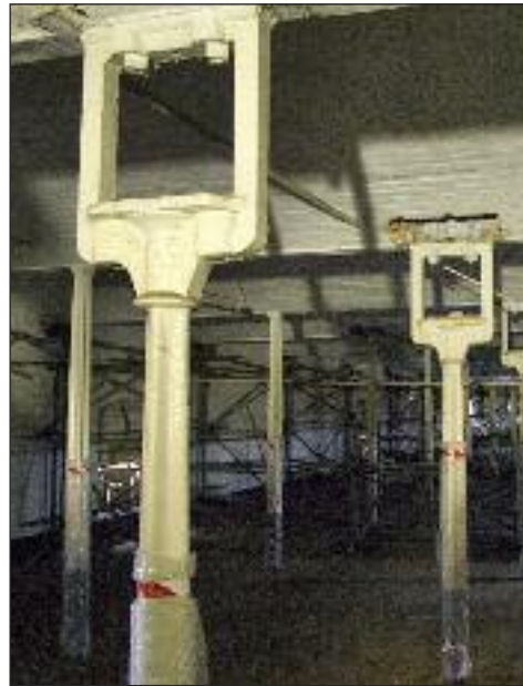
A supporting iron pillar in the mill, part of the first iron framed building in the world
