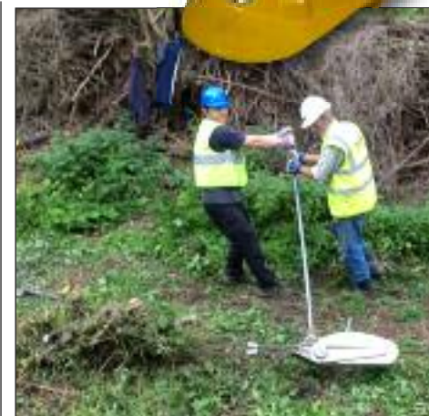
Andy Dady and Peter Cann using the 'Trifor' winch to remove a tree stump from the canal bed.
