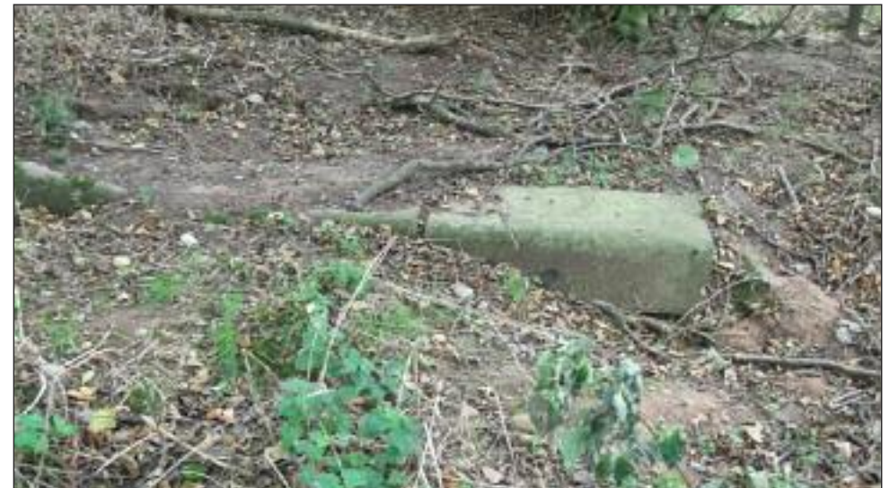
Buried stonework of the Swing Bridge
