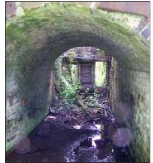
View under the bridge to the remains of the lock gate
