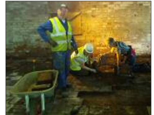
Removing the floor tiles from the small warehouse at Wappenshall
