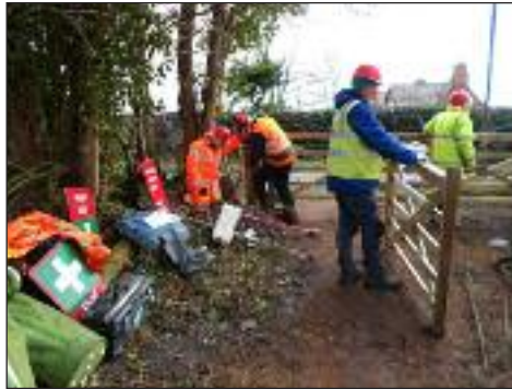
WRGies install new gates to the lane entrance
