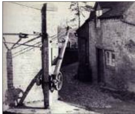
A crane at Uffington Wharf - part of Tom's length from his home in the basin in Shrewsbury
