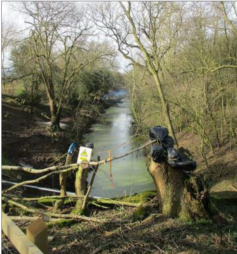
Slowly the canal emerged as clearance progressed
