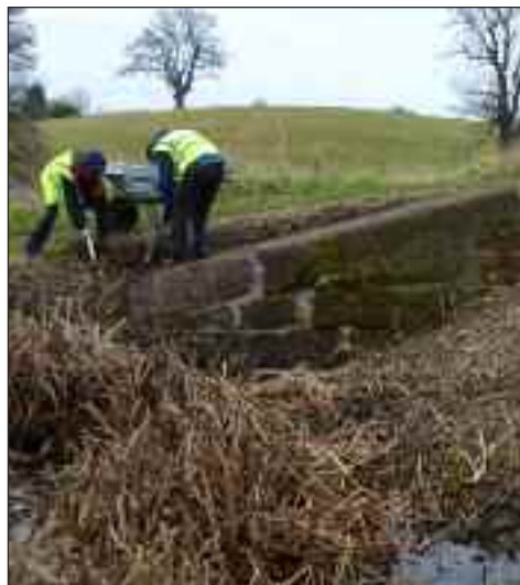
Terry and Ruth clearing the stonework at the entrance to Meretown Lock
