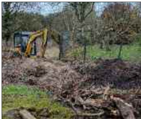
Digging out tree roots on the line of the canal
