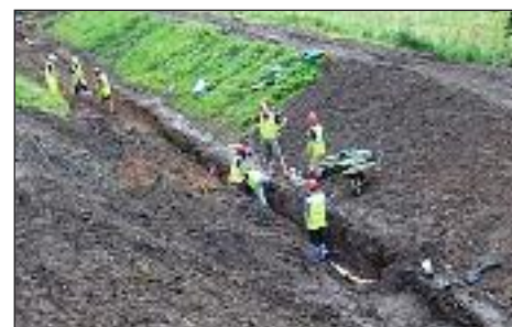
Installing the French Drain
