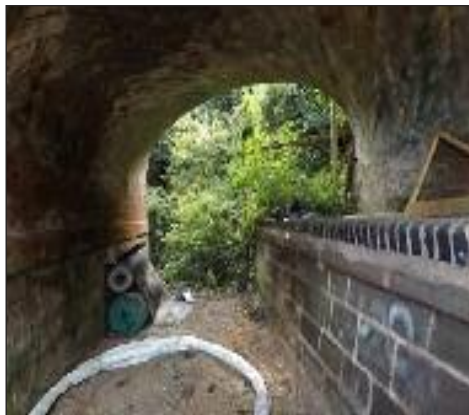
Re-pointed blockwork under the skew bridge No 10 at Forton
