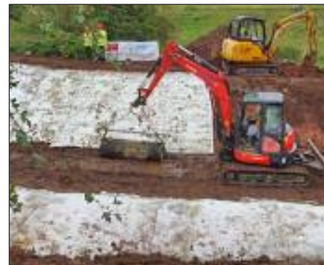
The WRG laying Bentonite lining at Forton prior to covering it in soil. This is now complete
