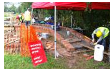
New access ramp to the footbridge over Meretown Lock
