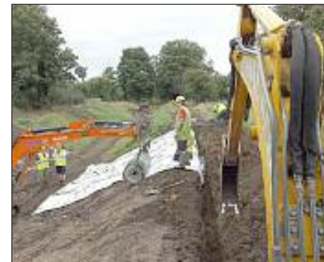
The WRG laying Bentonite lining at Forton prior to covering it in soil. This is now complete
