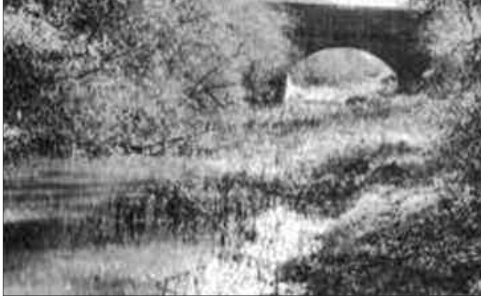
Bridge number 37 Widow's Bridge near Berwick Wharf on the Shredwisbury Canal
