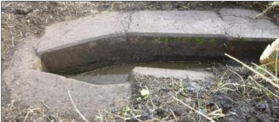
Is this the Tickethouse Lock bywash culvert?
