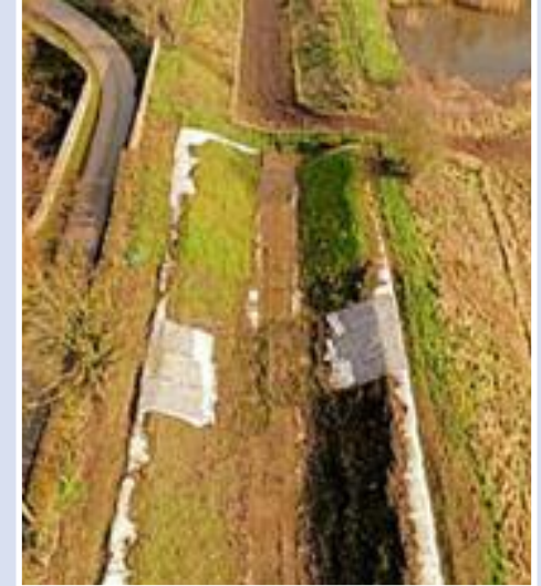
Forton restoration from above with some of the Bentonite lining still uncovered
