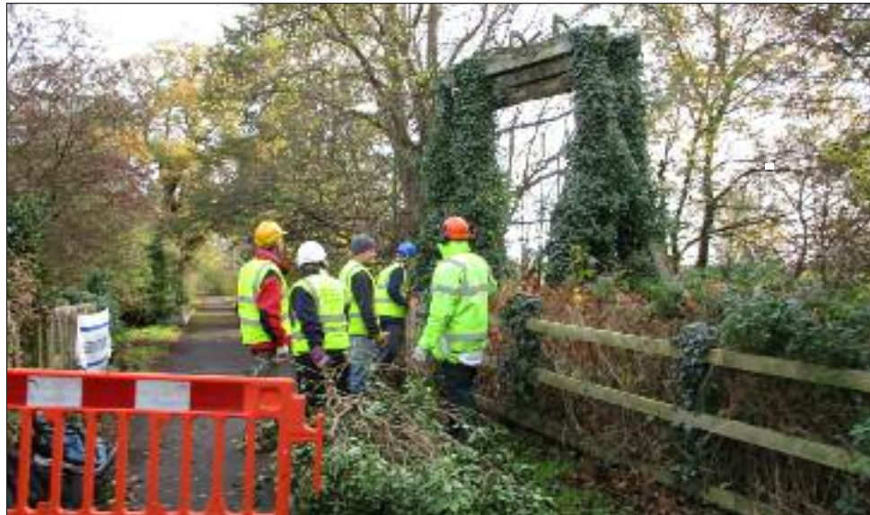
Clearing Hadley Park Lock area begins
