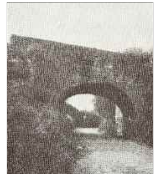
The aqueduct which carried the branch canal to Dawley
