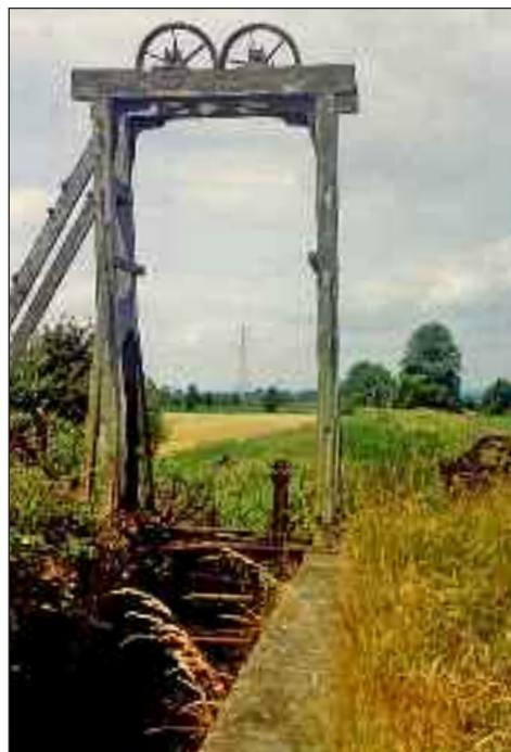
Turnip Lock No.3 on the Trench Arm in 1979
