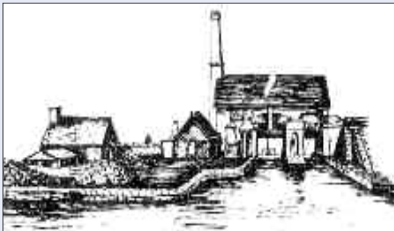
Old Wombridge Canal (incorporated in Shrewsbury Canal, 1793), basin and winding house.
