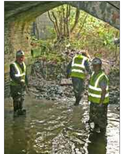
Working to clear water from the wharf under the Transhipment Warehouse
