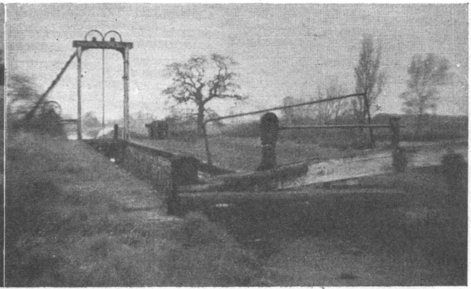
Britain Lock on the old Shrewsbury Canal. These locks, 51 feet long and 6 feet 4 inches wide, were the smallest in England.
